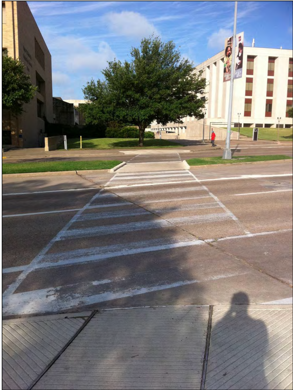
Exhibit 3. Existing east-west crosswalk, median nose, and street light pole on south side of N. Bizzell Street and Polo Road
